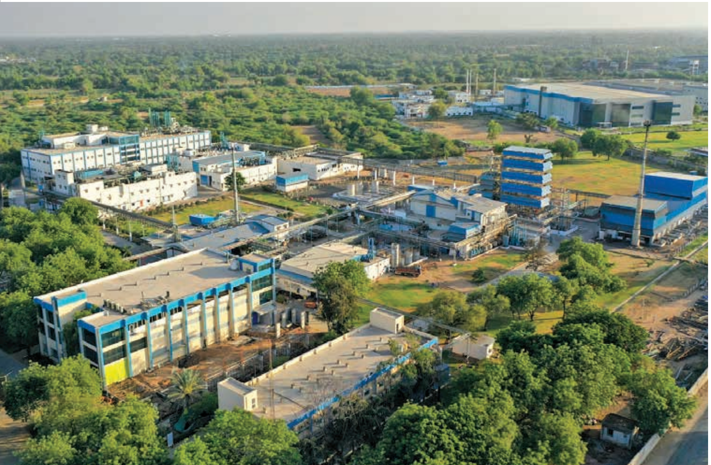
API plant, Karkhadi
