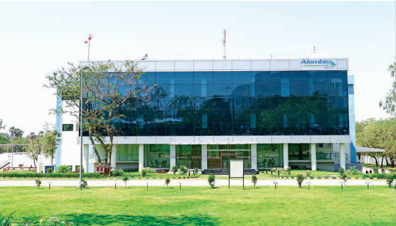
Oncology injectable and OSD plant (F2), Panelav
