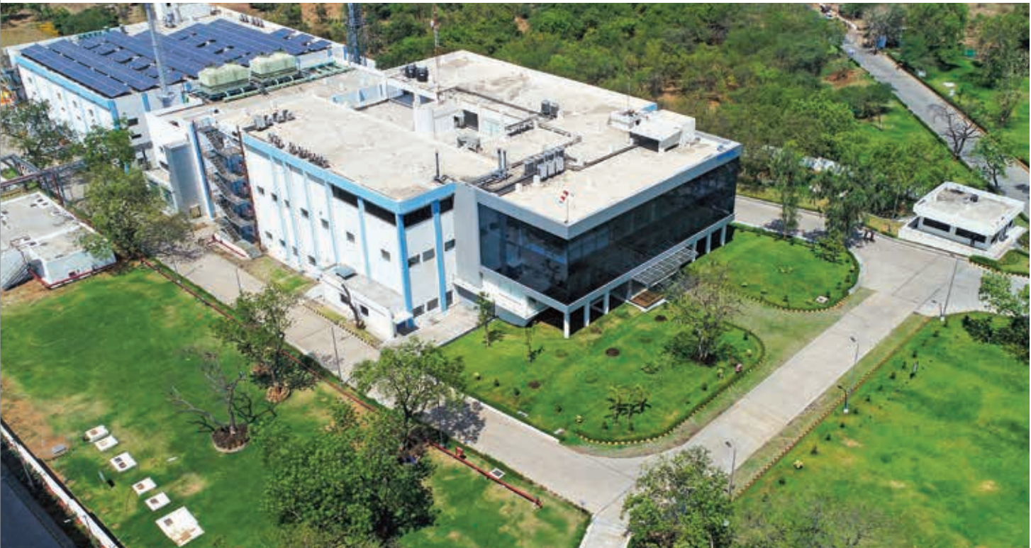
Oncology Injectable and OSD plant
